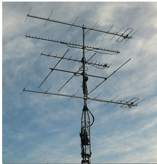
2 x 8el 144MHz LFA installed at G1MHU
