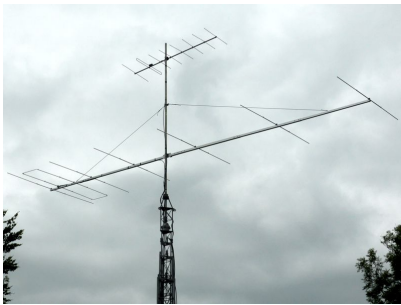
The 7el WOS installed are G2SJX
