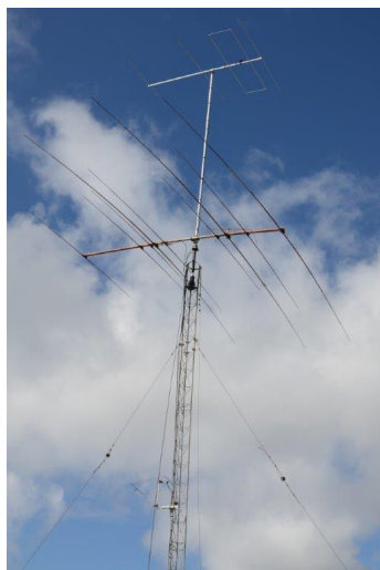
The 4 element 50MHz LFA-LN installed at ZD7VC
