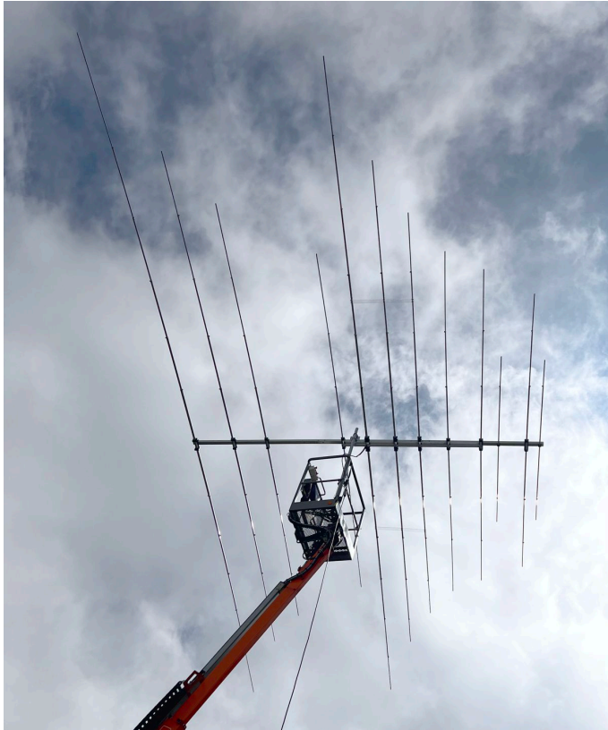
DXE 12-6 HF & 6m Yagi on 5.3m boom (20/17/15/12/10/6). The World's best 6 band HF & 6m Yagi 'full sized' Yagi - InnovAntennas
