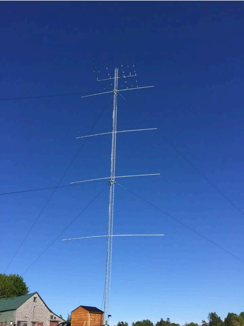
4 x 8el 11.7m 50MHz LFA-2 @ W2RE
