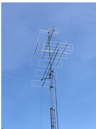
The 6el LFA-Q for 50MHz @ VE1PZ
