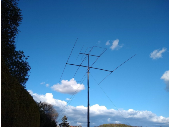
A High Gain 18MHz LFA Yagi
