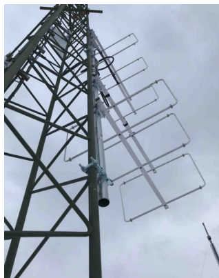
2 x 3el 144MHz LFA-Q (rear mount) installed at the SK3VHF Beacon site
